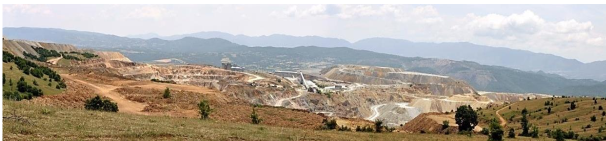
Figure 19 Mining landscape (Buchim mine)
